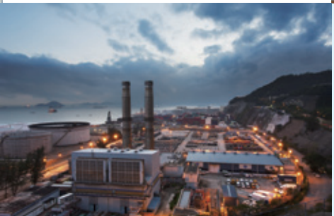
Power Electric supply
